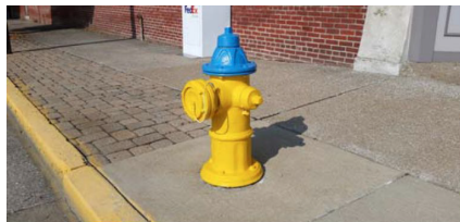
Blue Hydrant Top 1,500+ GPM Flow Capability with Quick Disconnect Fitting
